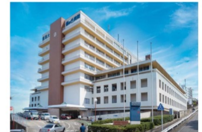
Showa Medical University Fujigaoka Hospital
