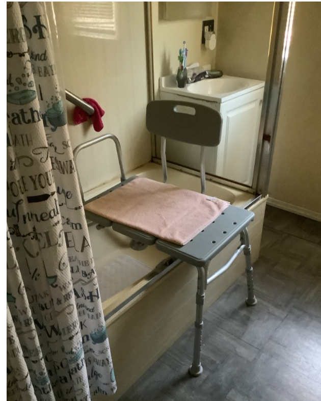
Post-Compass: Removed shower doors, replaced with curtain, added grab bar and tub bench for independent transfer
