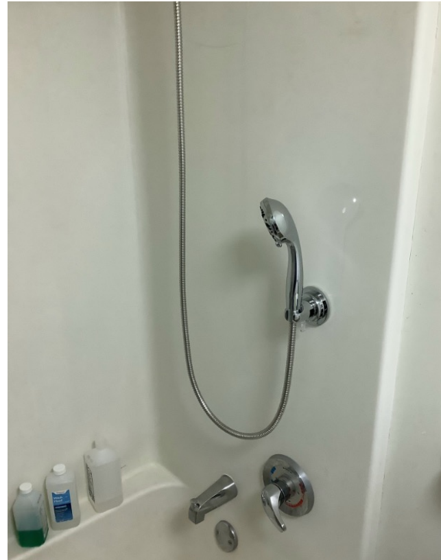
Post-Compass: Replaced tub bench (not pictured) and added hand-held shower head and suction cup holder
