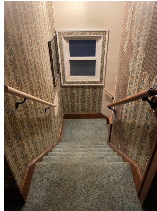
Post-Compass: Bilateral railing installed. Re-secured original railing.
